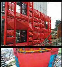
THE 13 consists of 4 levels of deep basement, and a 23-storey superstructure including 4 storeys of podium. Construction of the basement and superstructure was 14 months from excavation to topping out and completion of all late cast structures. The top-down method was chosen to help fast-track the superstructure, as using conventional building methods would have otherwise required an additional 8 months.
